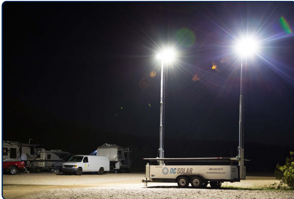
Figure 25 Light Towers in Use
