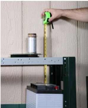
Measuring and marking before mounting the MNDC-X2 to the wall.
