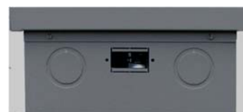
Battery box with 125 amp DC breaker. Remove only the inner knockout
