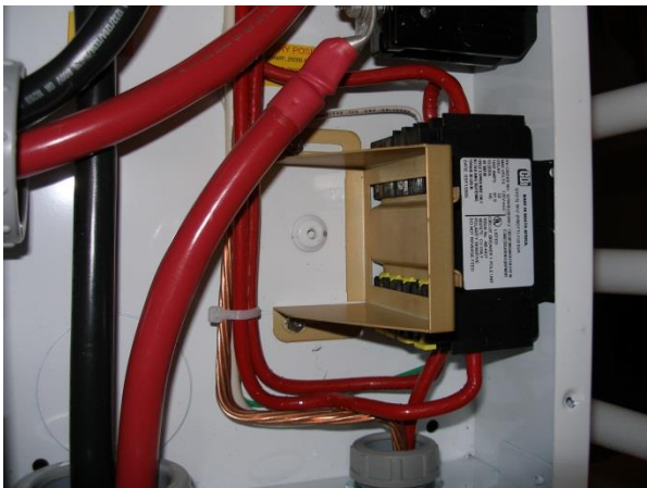
Din Rail mounted breakers
