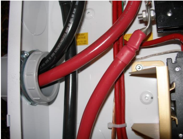
Wire exit to inverter
